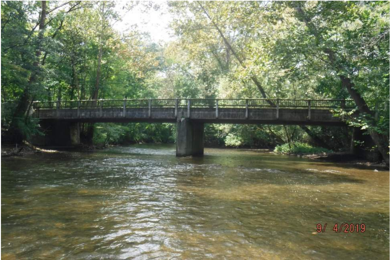
Existing York County Bridge No. 247
